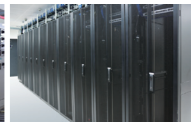
机箱机柜行业 Chassis cabinet industry
